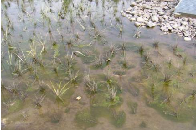
Figure 22 Algae growing on the filter media surface
