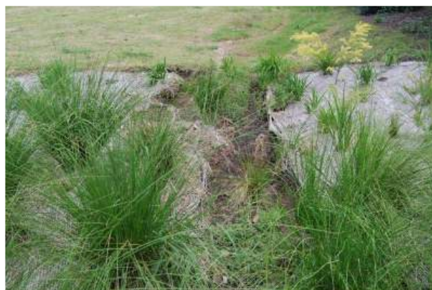
Figure 15 Erosion at the transition between wetland cells
