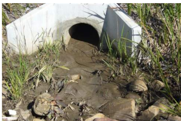
Figure 17 Sediment accumulated at an inlet
