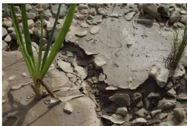
Figure 18 Examples of a bioretention surface that has been blinded with clay-like sediment deposition
