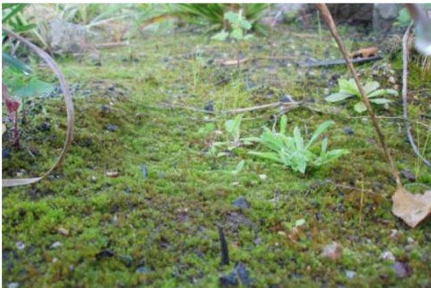
Figure 23 Moss growing on the filter bed surface
