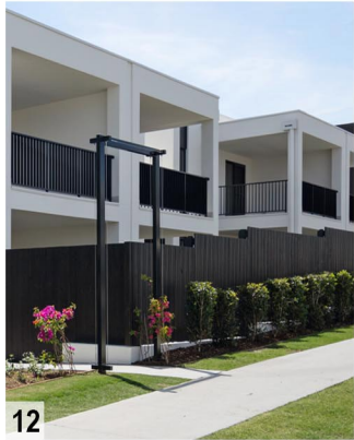
12. AZURE SAVILLE EDITION RICHLANDS - SEMI-TRANSPARENT FENCING ATOP RETAINING WALL
