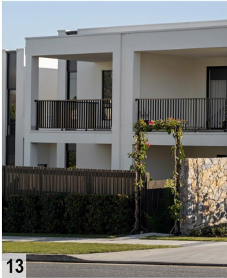
13. AZURE SAVILLE EDITION RICHLANDS - SEMI-TRANSPARENT FENCING ATOP RETAINING WALL
