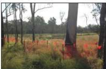
SIGNIFICANT TREE PROTECTION FENCING
