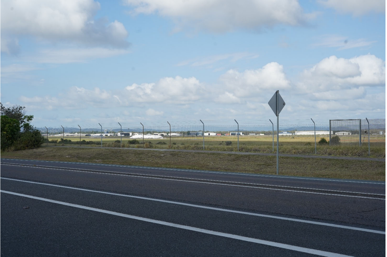
Plate 5-1 LCZ1 – representative image of current airport infrastructure (Photo: RPS)
