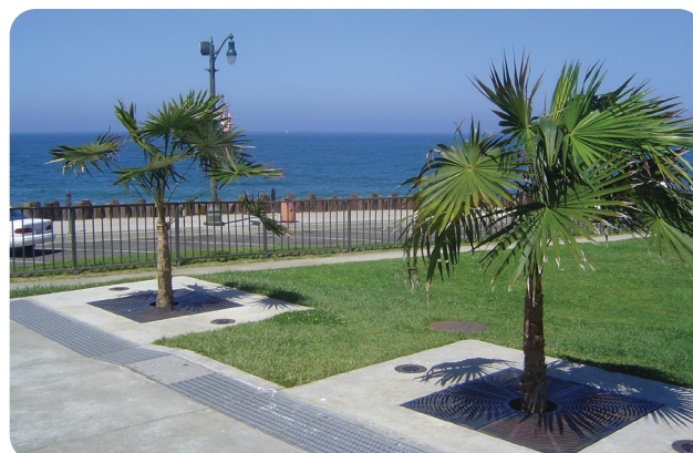
Figure 4: Filterra® tree pit – grated drain inlet
