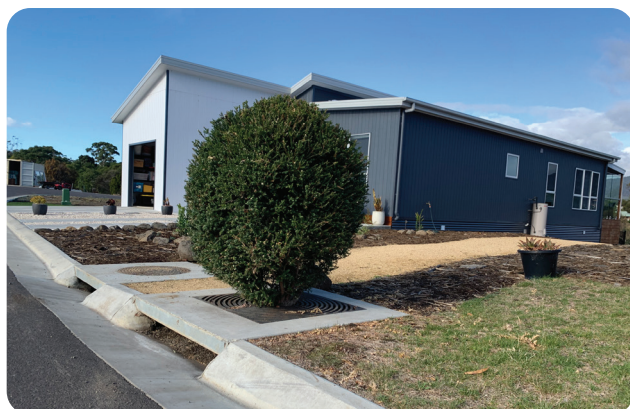
Figure 3: Filterra® tree pit – kerb inlet
