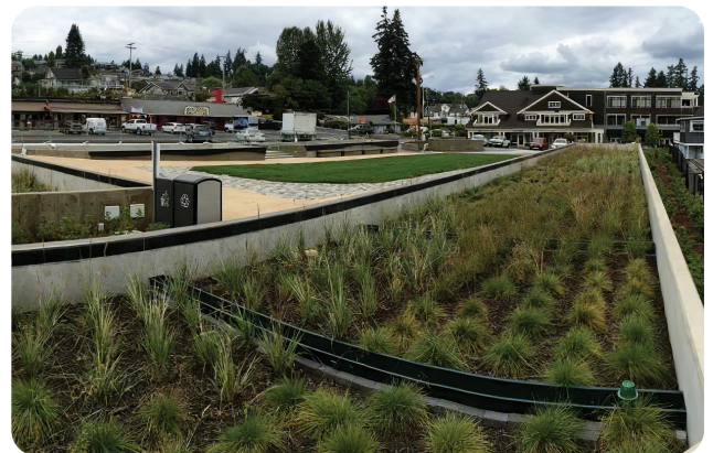
Figure 7: Filterra® bioscape – hard edging
