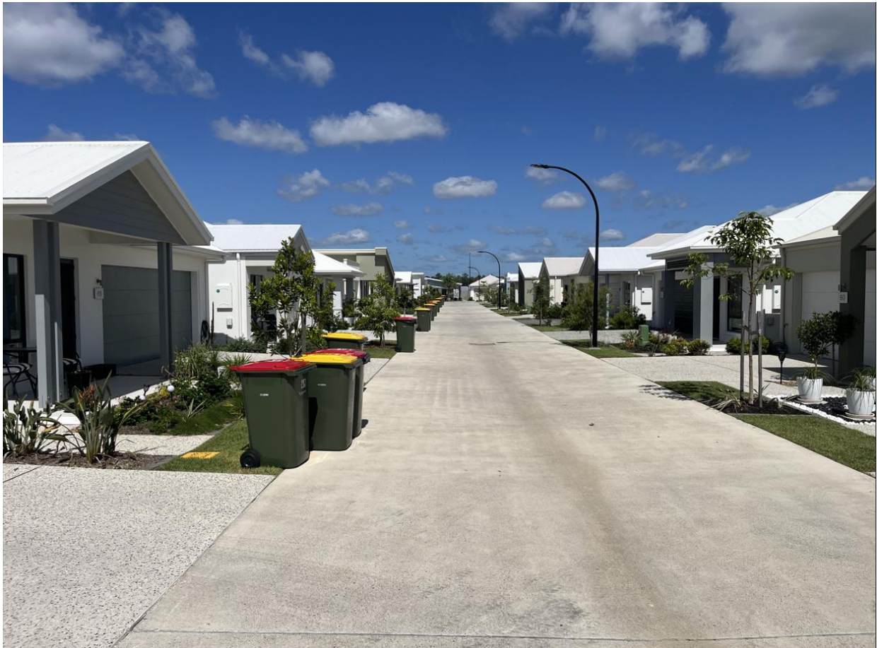
Figure 4 – Photo of Halcyon Coves showing bin placement (single sided) on collection day
