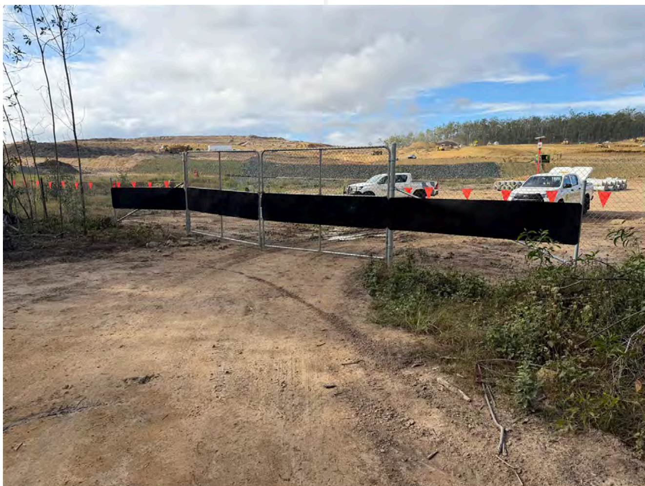
Photo: Fauna exclusion fence and access gates to be installed on either side of the bridge construction corridor.
