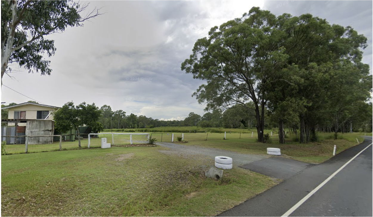
Figure 4: Site from Greenbank Road (Looking Southeast) (Source: Google Streetview)
