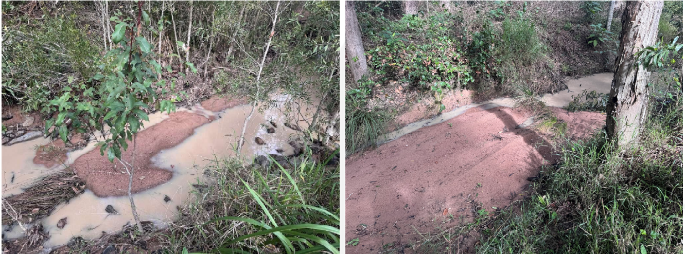
Photo set 6: Sediment deposits present along the mapped WWW within the eastern CA4 boundary vegetation.
