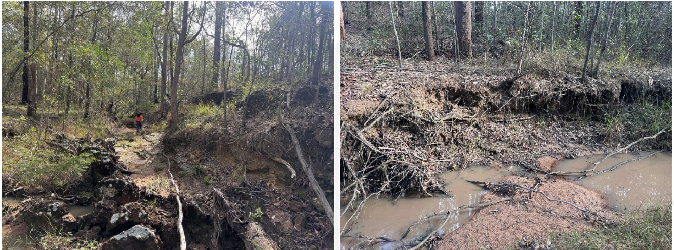
Photo set 10: Erosion present along the mapped moderate-risk WWBW south of the impact area.
