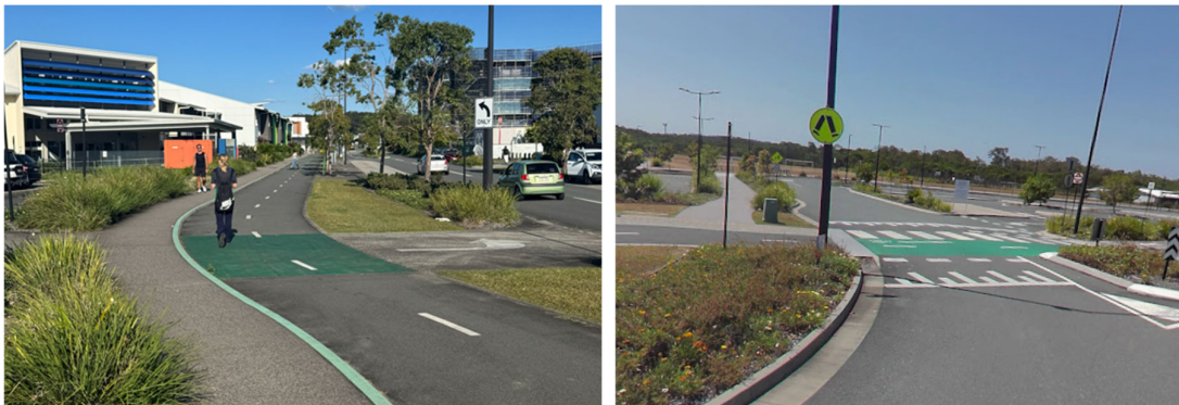
Photograph 2 & 3 – Separated Cycle Way on Baringa Drive and Raised Crossing
