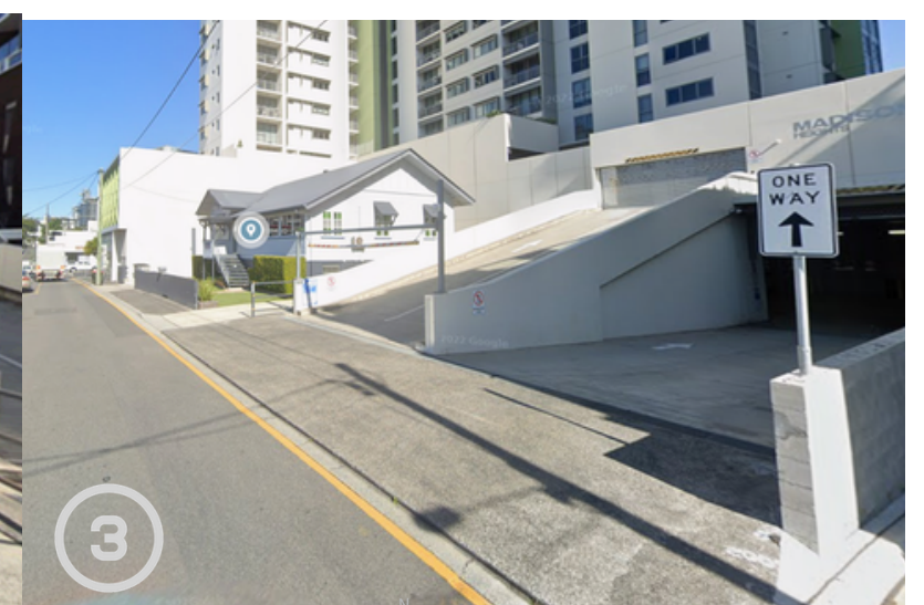
VIEW FROM NORTH EAST
