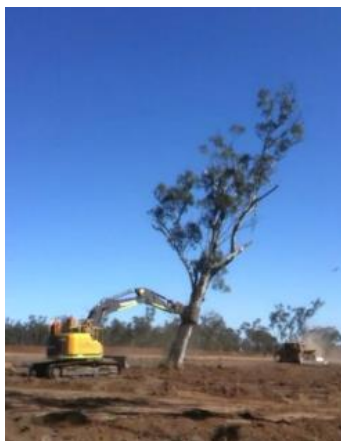
Photograph 2 Tree removal with use of grab attachment (DES, 2023)
