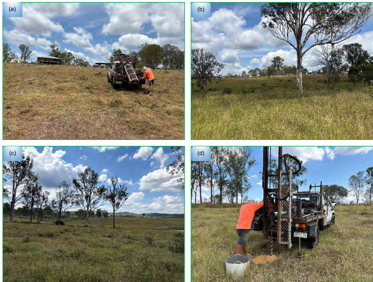
Figure 4: Selected Photographs of The Site
