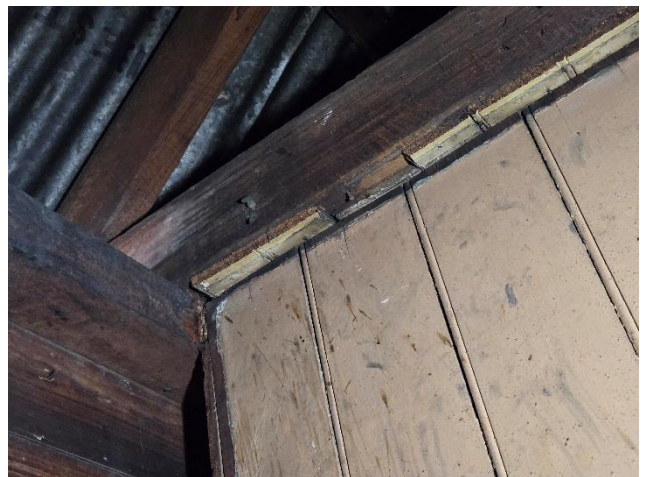
Walling and remnant vj boards adjacent.
