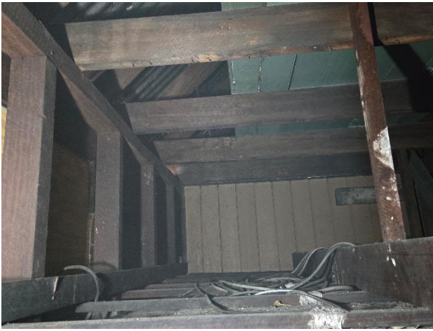
View above the existing ceiling.
