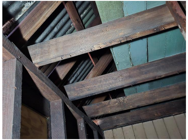
Floor framing above the ceiling showing remnant fixings of the original vj ceiling boards.
