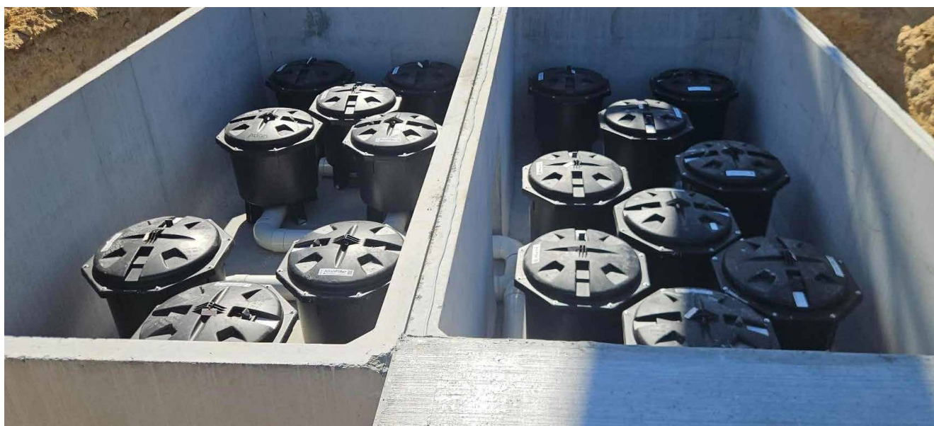
Figure 1 - AtlanFilters in a concrete chamber / vault
