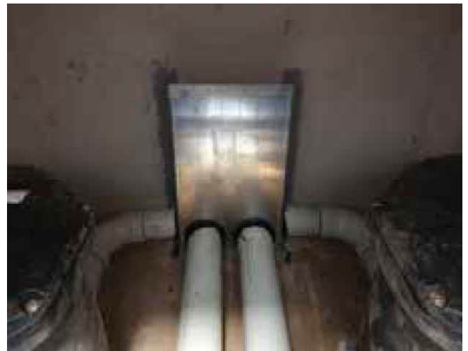
Figure 3 - Typical Outlet Weir Wall
