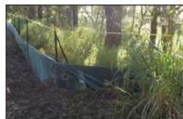
TREE PROTECTION & EROSION FENCE
