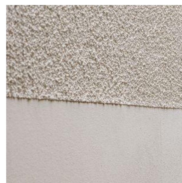
MASONRY RENDER FINISH MSN-1 & MSN-2 WALLS, CHANGE IN TEXTURE USED TO CREATE DATUM LINE
