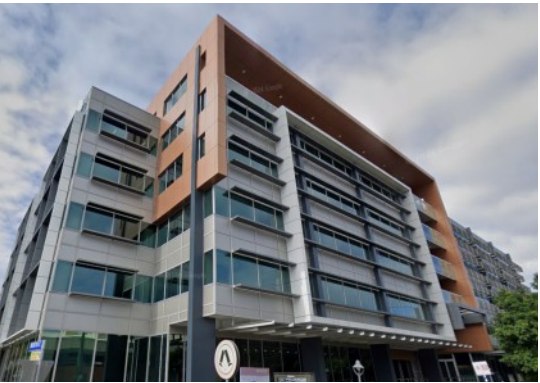
MUSGRAVE ROAD COMMERCIAL CONTEXT
