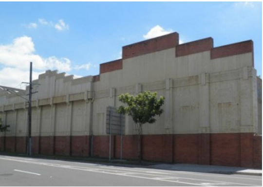
STEWART & LLOYDS FACTORY | LOCAL HERITAGE PLACE
