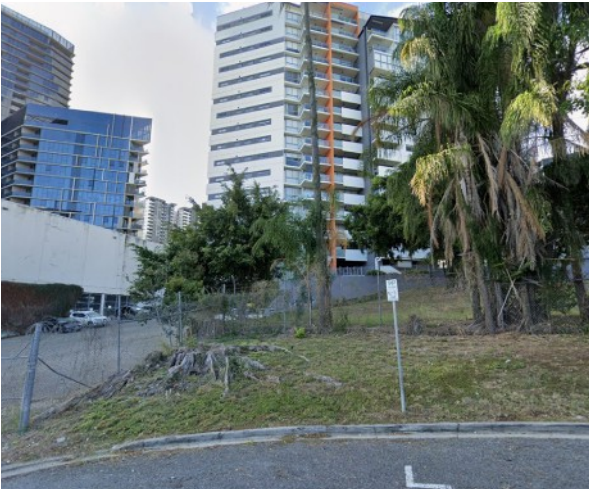
OXFORD STREET - LOOKING UP TOWARDS BOUNDARY ROAD - FUTURE CROSS BLOCK LINK
