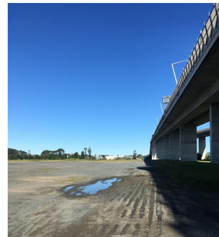
VIEW OF BRIDGE STRUCTURE FROM NEW ACCESS DRIVEWAY
