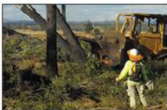
FAUNA SPOTTER DURING TREE CLEARING
