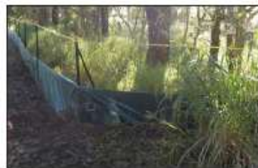
TREE PROTECTION & EROSION FENCE
