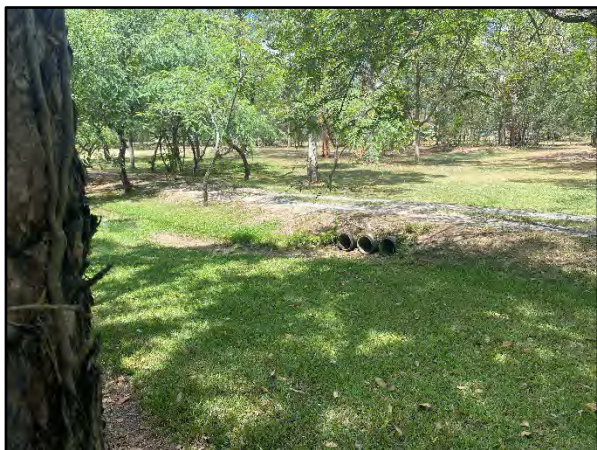
Plate 13 Modified drainage channel located to the southwest of the subject site
