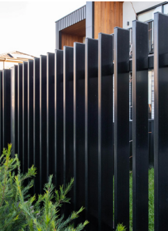
1.8m Security Fenceline
