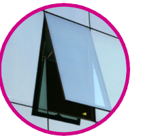
5.0 CURTAIN WALL GLASS WITH OPERABLE WINDOWS
