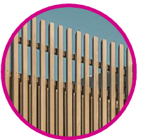
6.0 ALUMINIUM BATTEN SCREENING COPPER ANODIZED
