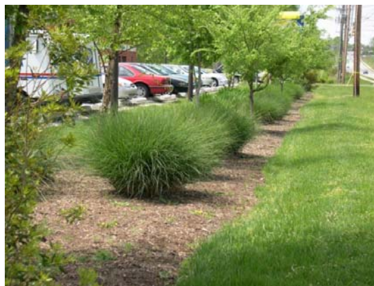
Photo 7 - Bioretention Swale
