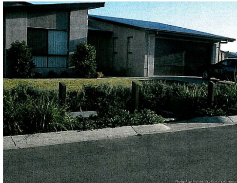
Photo 9 - Bioretention Basin/Garden
