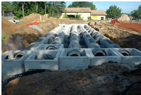
Photo 2 - Underground Detention Tank
