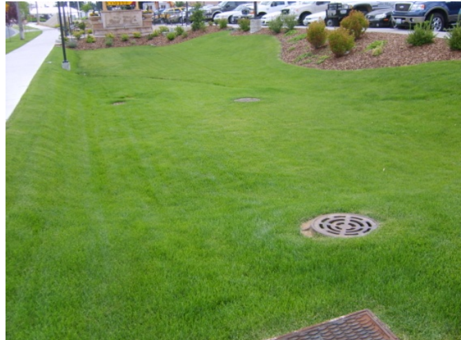
Photo 6 - Buffer Strip & Swale
