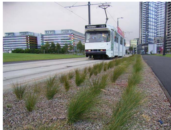
Photo 23 - Median Biofiltration
