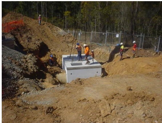
Photo 14 - Example of a Humeguard (under construction)
