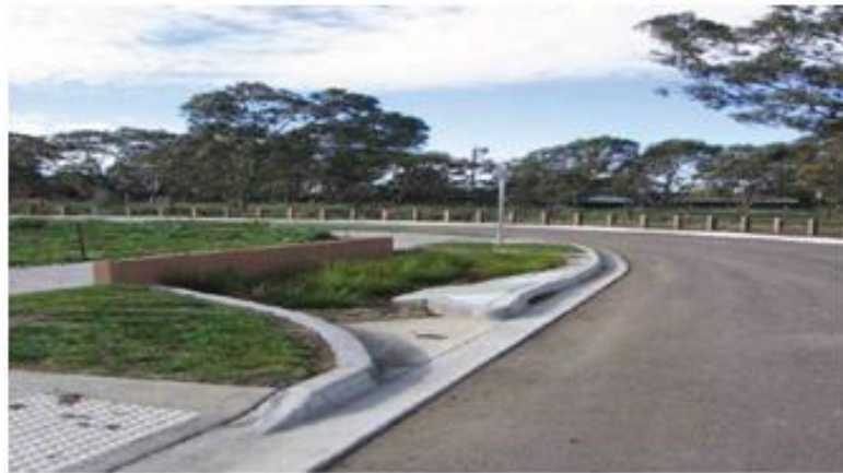
Photo 21 - Stormwater Pit downstream of Bio-retention Garden
