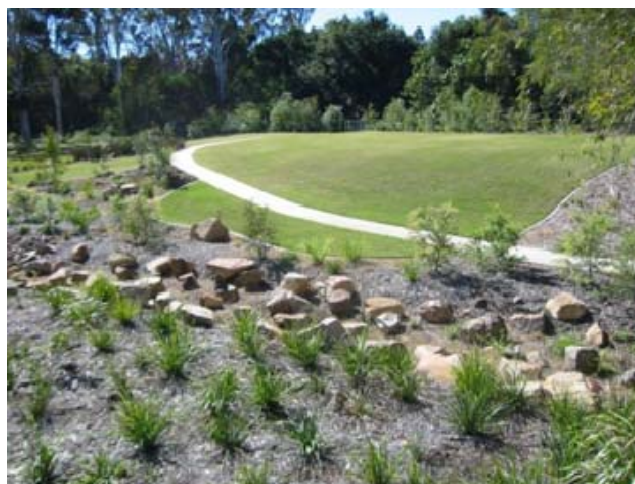
Photo 10 - Bioretention Basin
