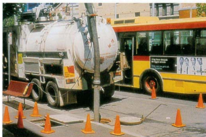
Photo 16 - Induct Truck at a Humeguard GPT during waste removal
