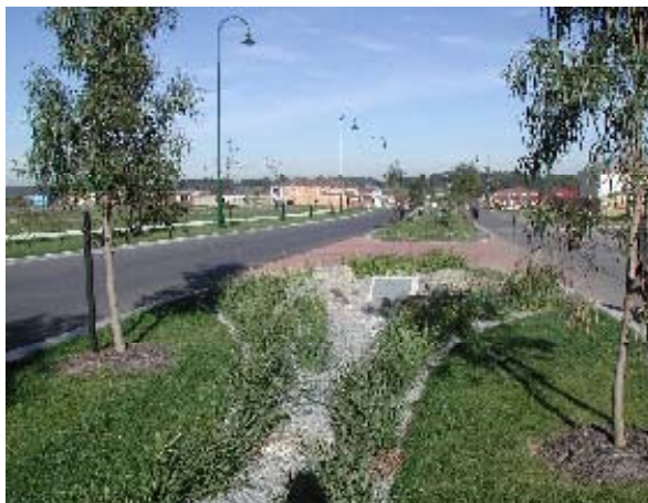
Photo 22 - Median Biofiltration
