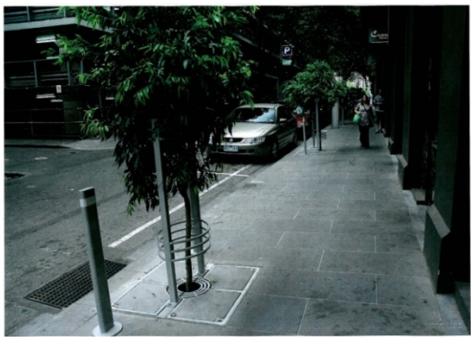
Photo 8 - Bioretention Pod
