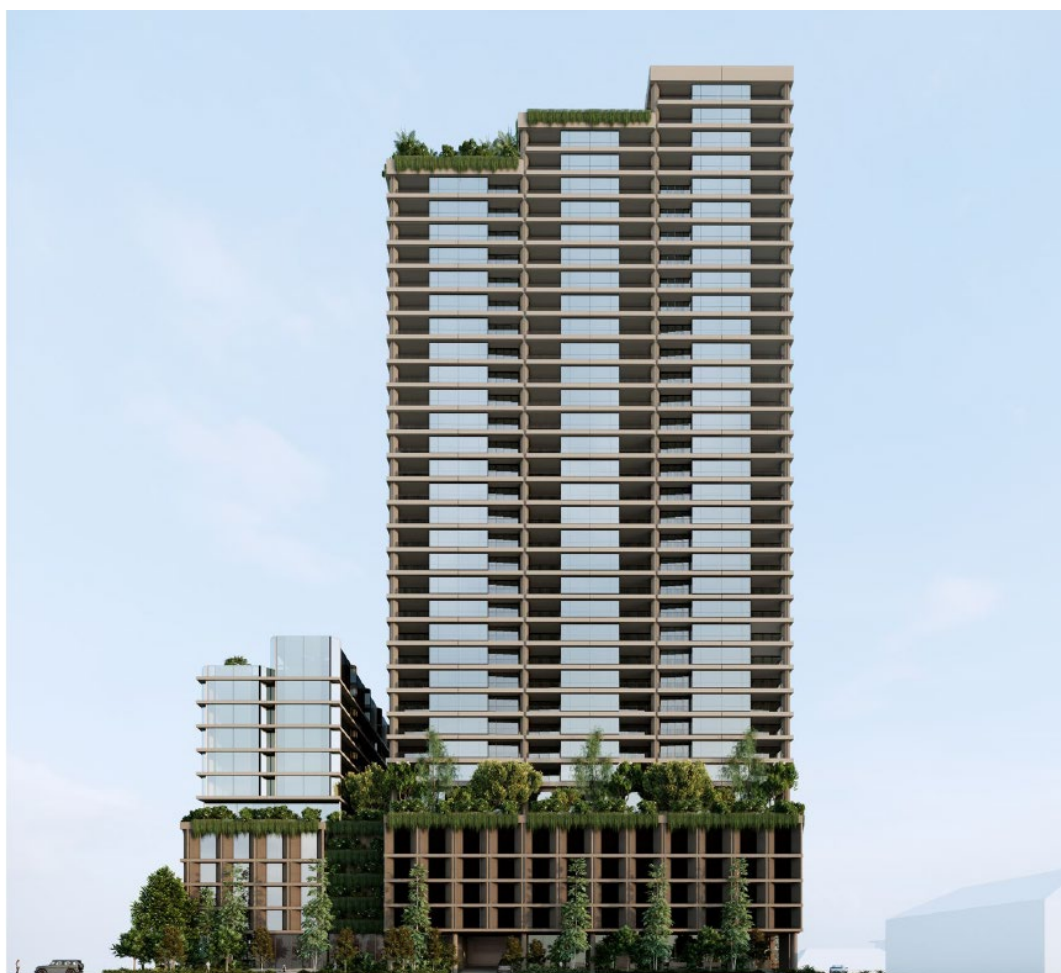
Figure 23 – Tower 2 view from Mark Lane
