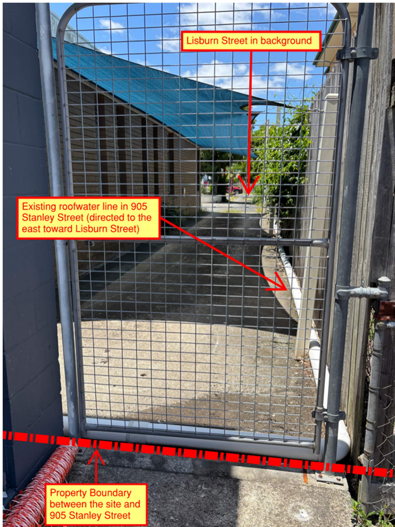
Figure 4.4 Existing Roofwater line that exists within 905 Stanley Street (photo taken on the eastern site boundary in an eastern direction toward Lisburn Street. Note that the existing roofwater line is laid above the ground)
