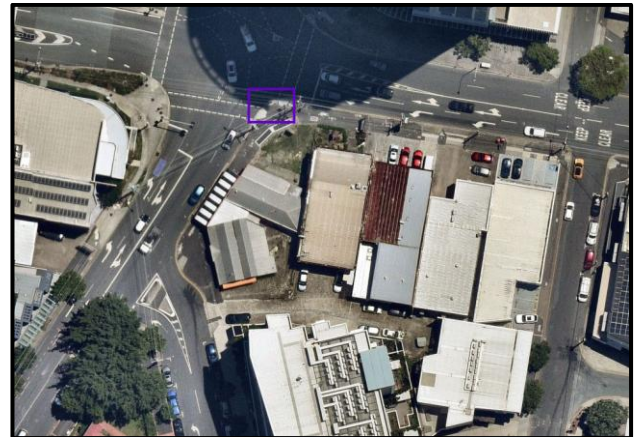
Figure 3: Aerial Imagery of Existing Gully Pit Location
