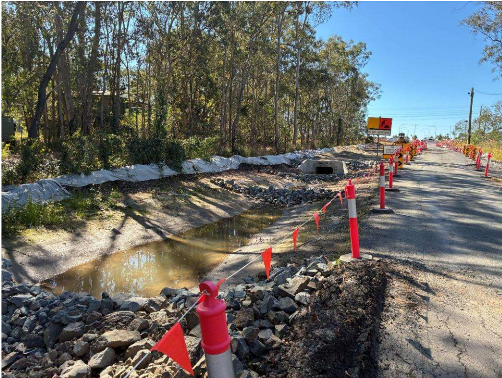
Figure 3-2 Existing constructed stormwater and table drain on Leanne Court (Source: WT 2025)
