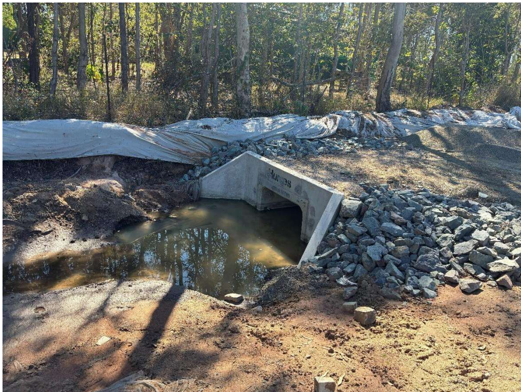
Figure 3-3 Existing constructed stormwater on Leanne Court (Source: WT 2025)
