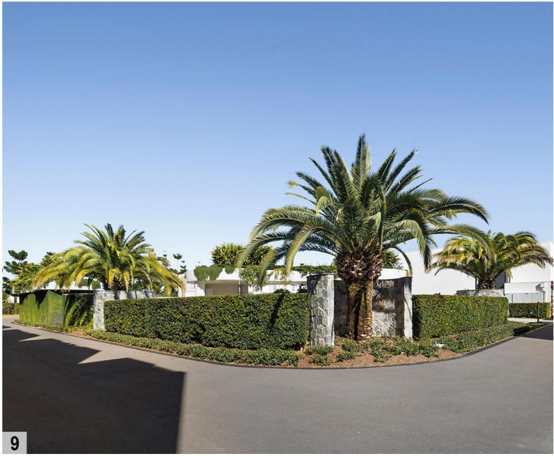
9. AZURE THE TERRACES MANGO HILL - COMMUNAL OPEN SPACE VIEWED FROM INTERNAL ROADWAY, FULLY SCREENED WITH VEGETATION FOR PRIVACY
