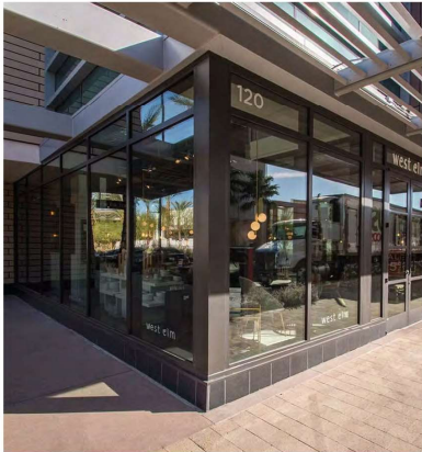
Shopfront Glazing with Black Framing
