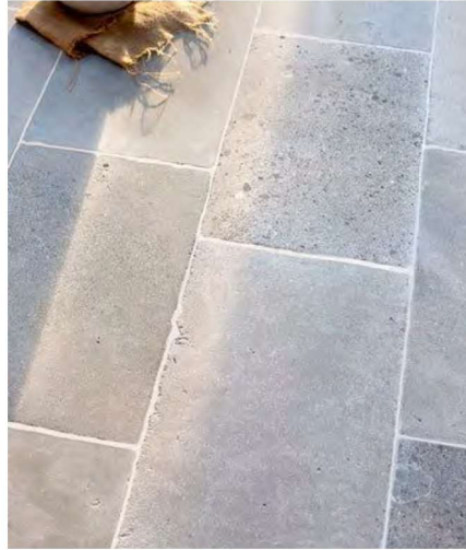
Entry foyer: Stone or concrete pavers
