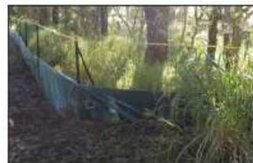
TREE PROTECTION & EROSION FENCE
