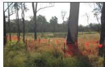
SIGNIFICANT TREE PROTECTION FENCING
