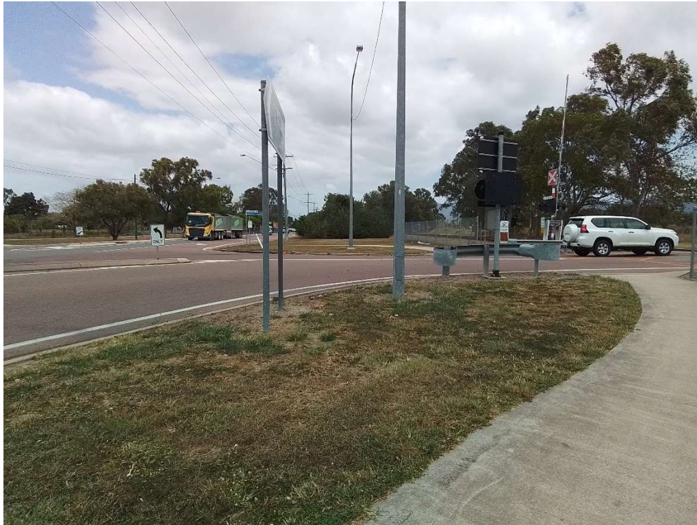
Image B – The Abbott Street/Lakeside Drive intersection looking south
