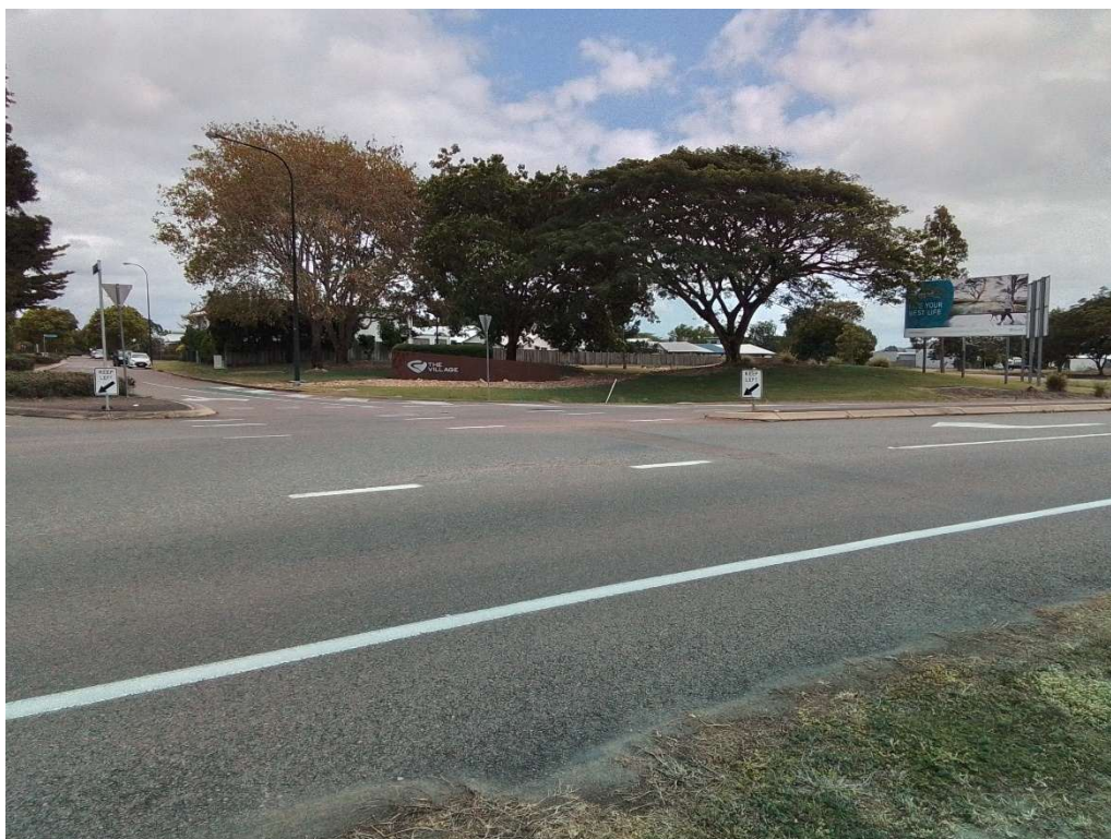
Image A – The Lakeside Drive/Riveredge Boulevard Intersection looking west
