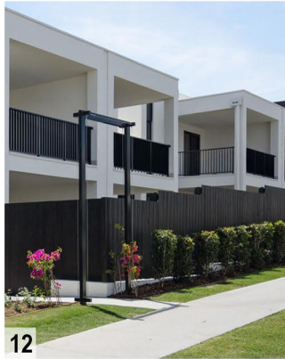
12. AZURE SAVILLE EDITION RICHLANDS - SEMI-TRANSPARENT FENCING ATOP RETAINING WALL
