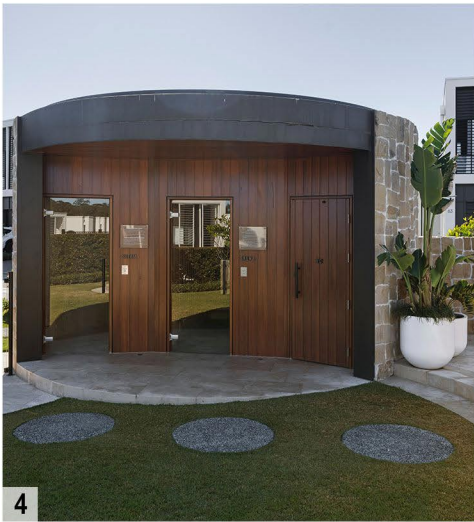
4. AZURE SEASONS BROOKWATER - STEAM ROOM SAUNA AND GYMNASIUM
