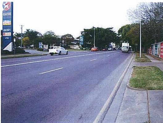
Figure 2.3: Kingsford Smith Drive Adjacent to Site (facing east)
