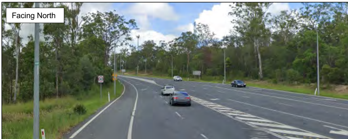
Figure 2.5 – Formation of Waterford Tamborine Road Adjacent to the Site
