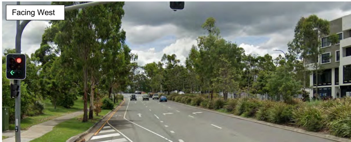
Figure 2.4 – Formation of Yarrabilba Drive Adjacent to the Site
