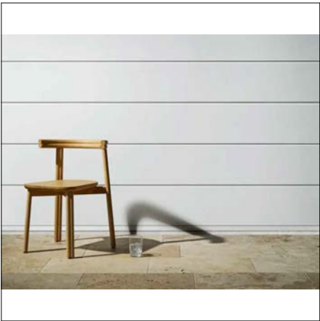
PAINTED FC (FIBER CEMENT) HORIZONTAL CLADDING JAMES HARDIE - STRIA (325mm)
