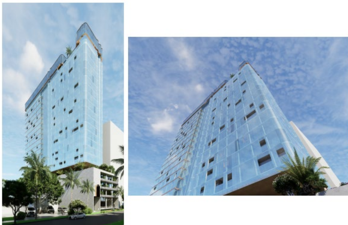
Figure 5: Tower Facade (SheltaCo)
