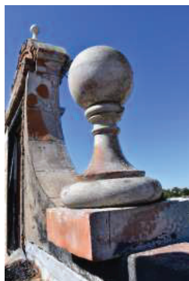
Figure A2.14 Terracotta parapet detail
