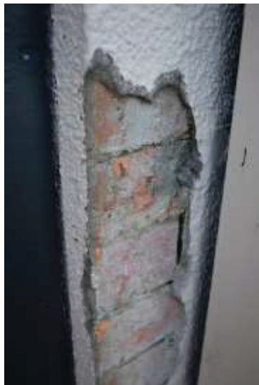
Figure A2.7 Rendered brickwork
