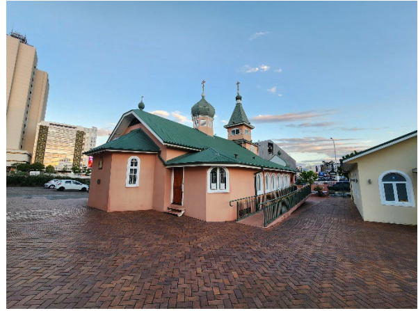
Picture 21 Rear elevation of the cathedral
