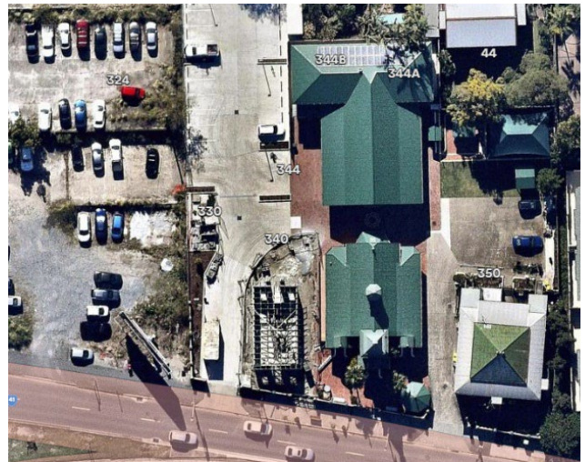
Picture 11 Aerial image of the site in July 2016 and the new baptistery is in the process of being constructed
