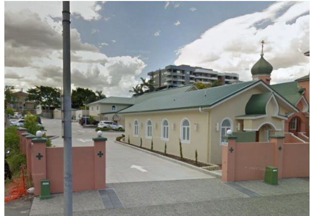
Picture 13 The new baptistry in March 2017
