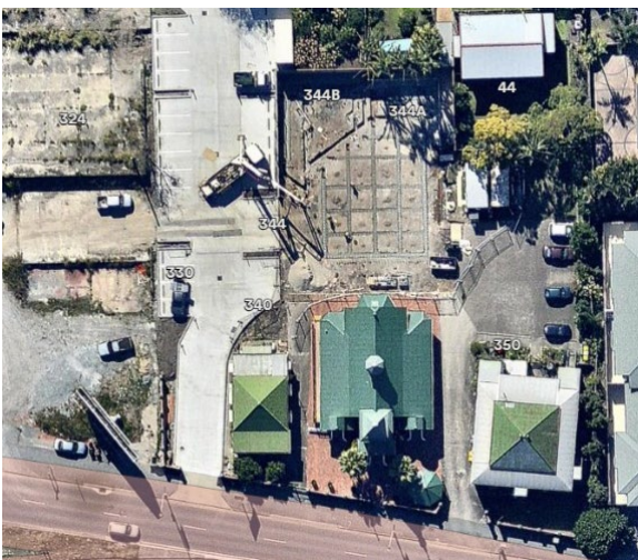
Picture 10 Aerial image of the church showing the demolished hall to the rear of the site in July 2015
