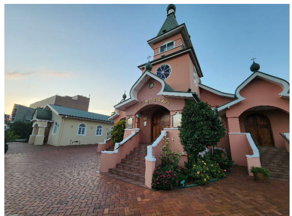
Picture 23 The primary elevation of the cathedral
