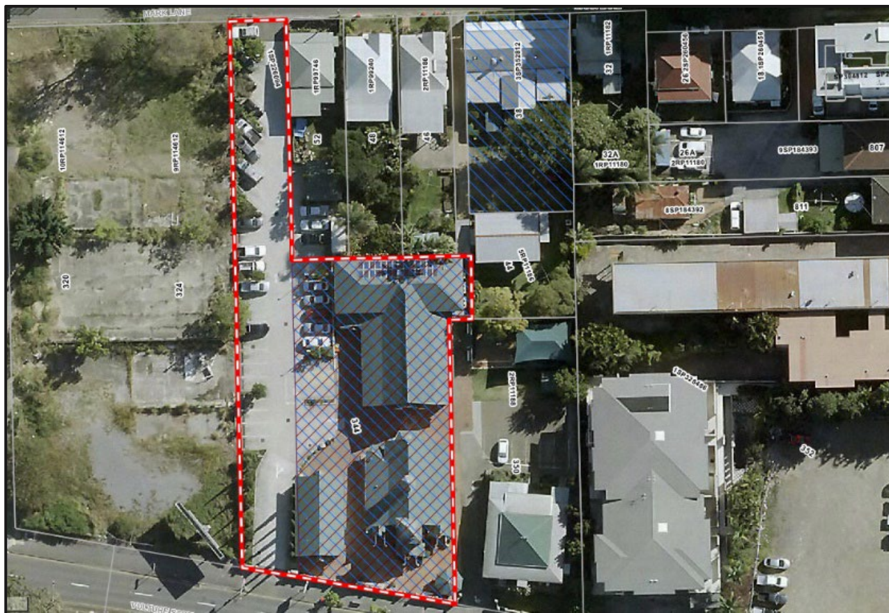
Figure 3 Aerial photograph of the cathedral lot (red outline) and the heritage curtilage of the State Heritage Place.
