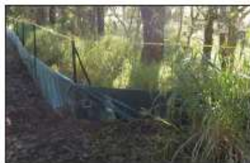
TREE PROTECTION & EROSION FENCE
