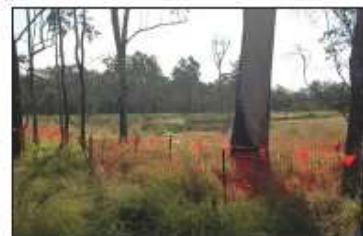
SIGNIFICANT TREE PROTECTION FENCING
