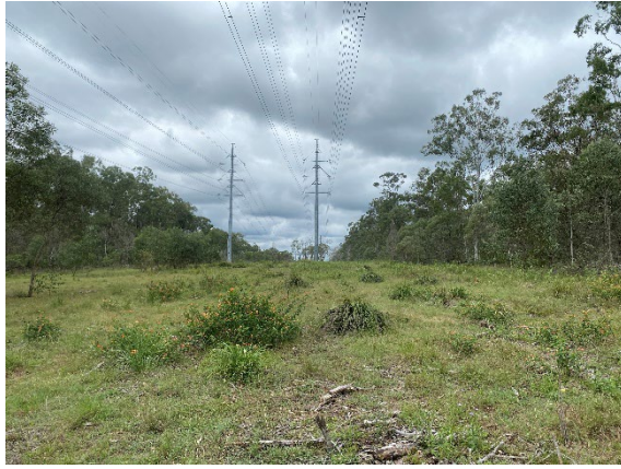
Photograph 3.3 VHC 40.4 within BAU 3
