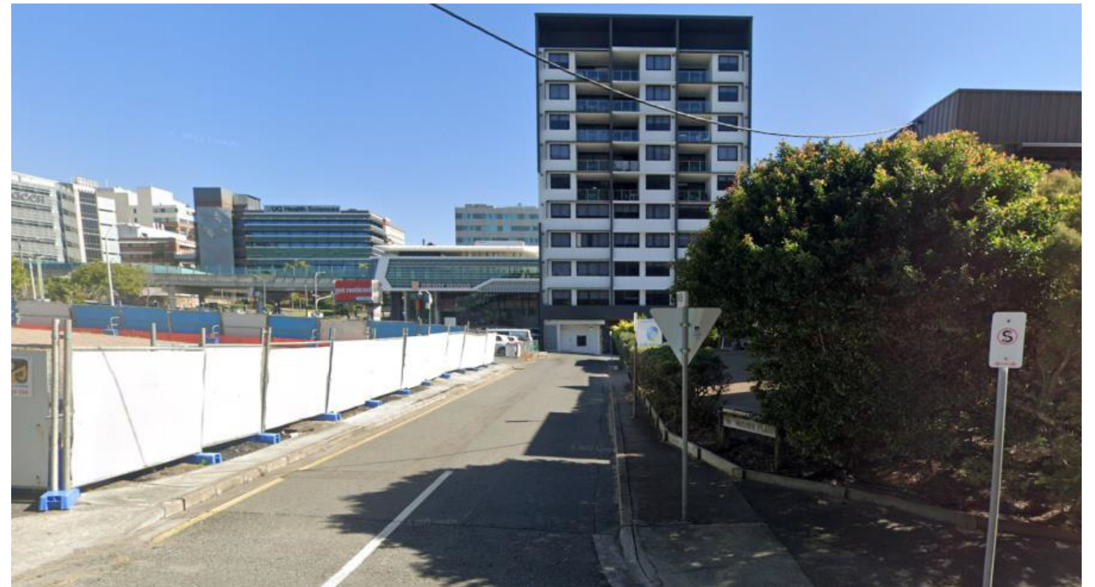
WALDEN LANE SITE: EXISTING CONDITION
