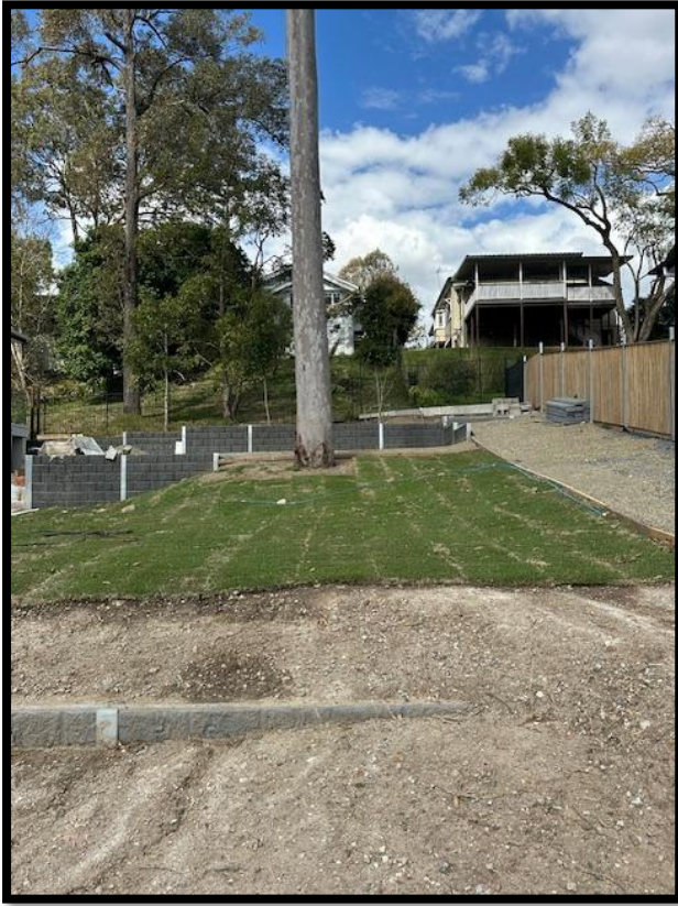
Plate 10: Turf being laid.
