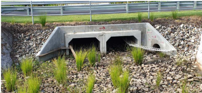
Image: A culvert with dry ledges
