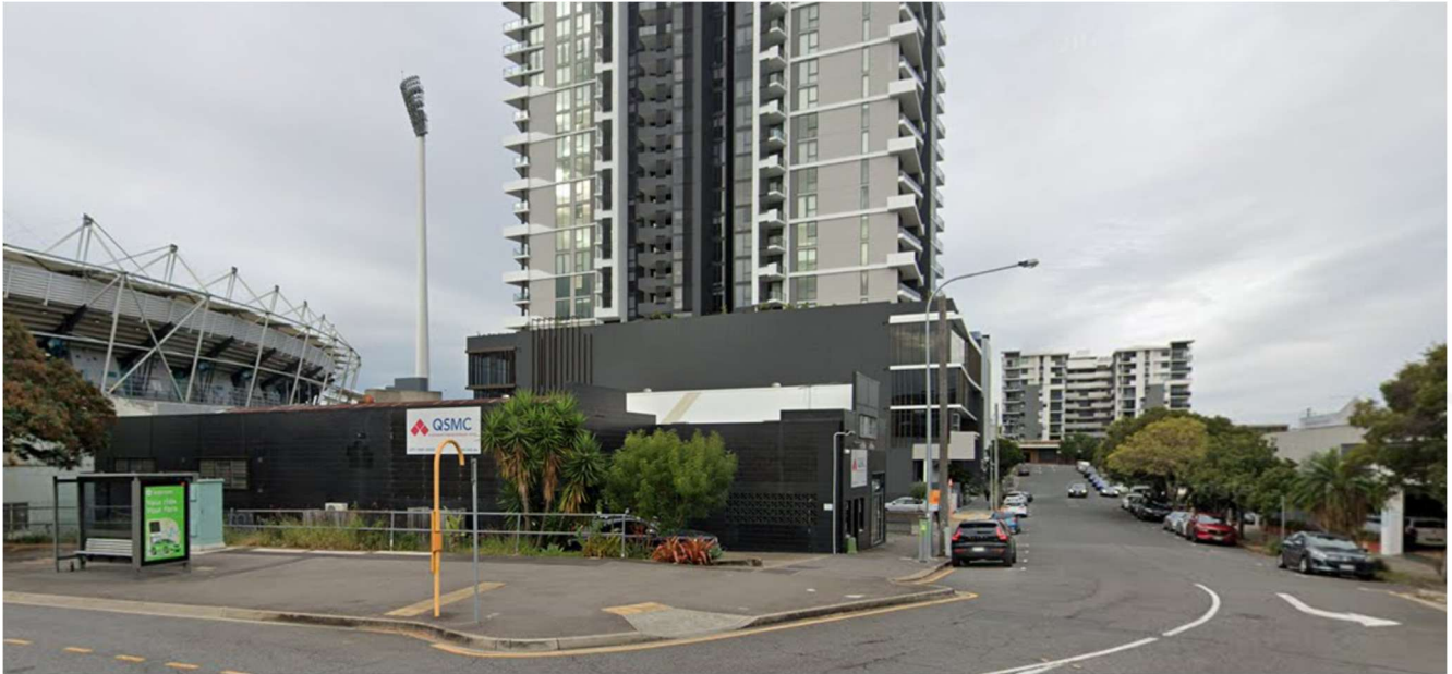
Photograph 5: Intersection of Trafalgar Street and Jurgens Street, viewing towards the subject site, with Silk 1 in the background (Source: Google Maps 2022)
