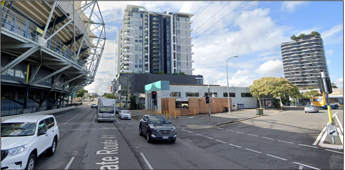
Photograph 3: Intersection between Stanley Street and Jurgens Street, viewing towards subject site with Silk 1 in background (Source: Google Maps 2022)
