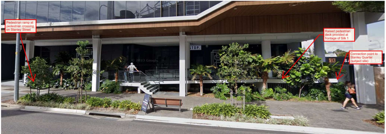
Figure 5: Silk 1 frontage to Stanley Street, showing elevated pedestrian deck which will eventually link in with the pedestrian plaza within Stanley Quarter.
