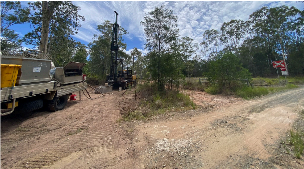
Photograph 1: General site conditions (view looking northeast towards borehole BHB and rail line)
