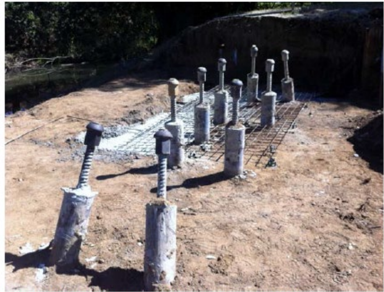
Photographs 2 and 3: Micropile installation equipment and view of micropiles installed in a bridge abutment
