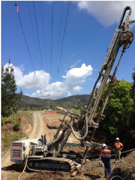
Photographs 2 and 3: Micropile installation equipment and view of micropiles installed in a bridge abutment
