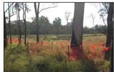
SIGNIFICANT TREE PROTECTION FENCING
