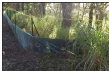
TREE PROTECTION & EROSION FENCE
