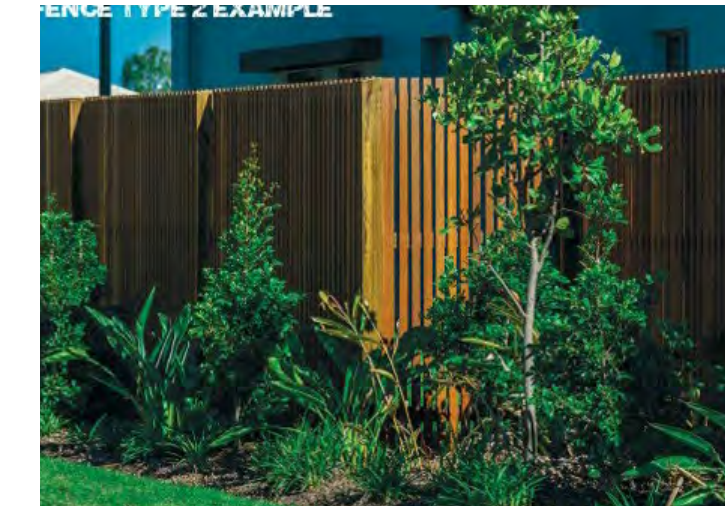
1.8m Corner Lot & Feature Fencing – 50% Transparency
